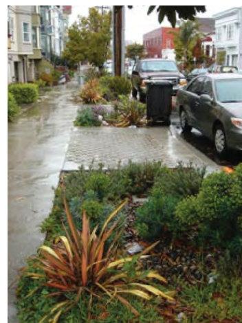
Figure 80. Storm water source controls like these rain gardens reduce pollutant run-off.
