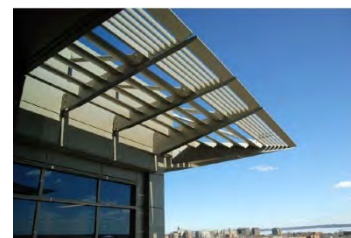
Figure 64. Sun shading devices reduce lighting and cooling demands and protect the building envelope from pre-mature aging.
