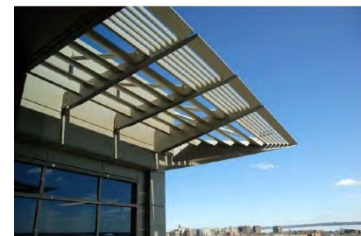
Figure 64. Sun shading devices reduce lighting and cooling demands and protect the building envelope from pre-mature aging.
