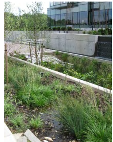
Figure 79. Weirs and check-dams help to slow the flow of water and facilitate infiltration.
