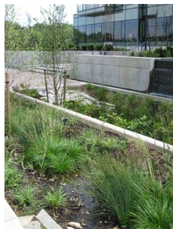
Figure 79. Weirs and check-dams help to slow the flow of water and facilitate infiltration.
