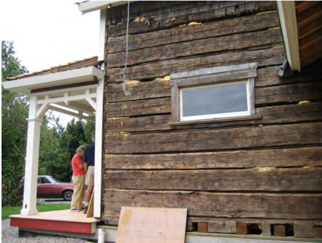
Leaf Residence showing the square hewn logs beneath the shingle siding
