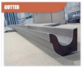
Profile of new wooden gutter sourced from Standard Building Supplies.
