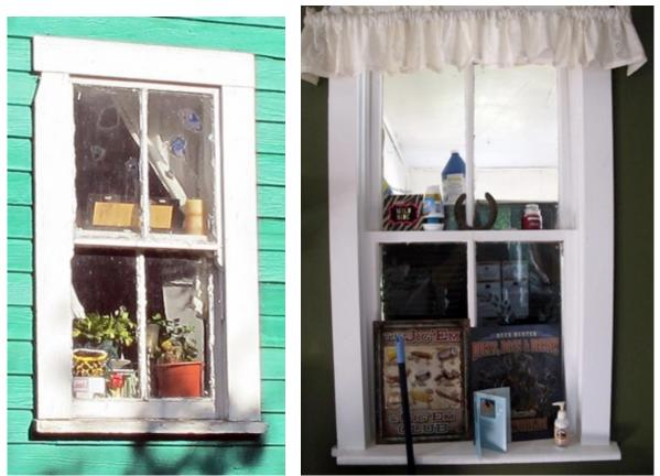
Left: West Elevation, original pre-1907 window with 2-over-2 double-hung wooden sash. Right: North Elevation, interior of pre-1907 window.
