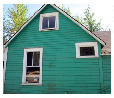
Left: North Elevation of 1896 House. Original 1896 window frame to left; window to right blocked-in when the stairs were built, and new window installed. Attic window presumably installed at the same time.
