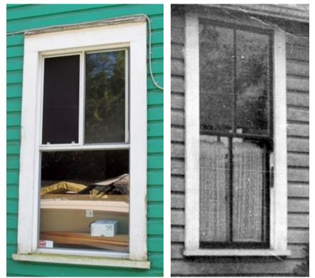
Left: North Elevation, 1896 window with replacement aluminum sash. Right: Original appearance of 1896 windows.
