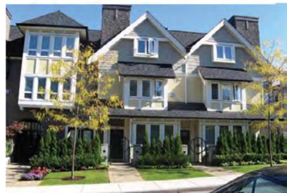
Variation and consistency is achieved by breaking the facades into a series of intervals
