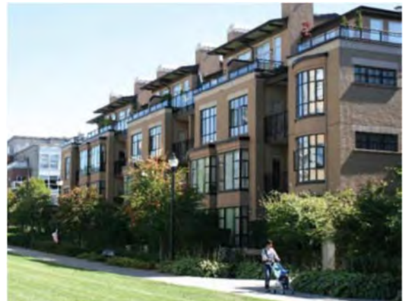
Massing contributes to the pedestrian experience through vertical setbacks, upper storey step-backs, and varying roof planes
