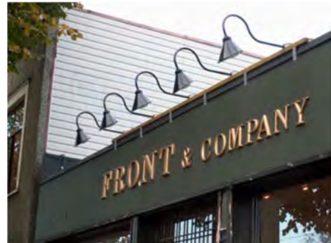
Externally lit building signage
