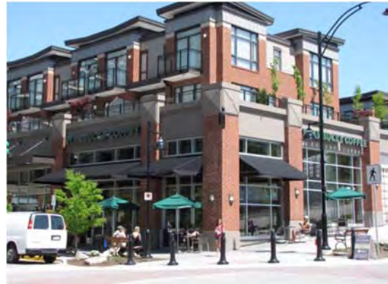
Glazing, weather protection, and shop front cornices on storefronts
